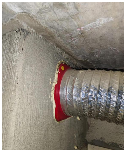
图 9.2.2-2 止回阀漏烟修补
